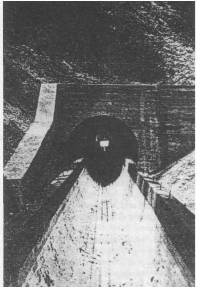
Fig. 12.3 Egg-shaped form of log flume
